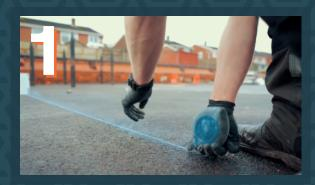
Clean application area thoroughly by removing all sand, dirt, chemicals and oily substances, measure & mark.
