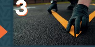
Remove the packaging and carefully place the marking onto the prepared surface, with the glass-coated top facing up. Position as accurately as possible and cut to size if required.
