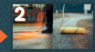
Using a suitable propane torch, remove any moisture present and preheat the area prior to treatment. Use a suitable primer on non-asphalt and aggregate rich surfaces. Allow primer to dry.
