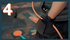
Heat the marking using a suitable propane torch keeping the flame approximately 20-40cm from the marking. Do not concentrate the heat in one area. Instead, heat with an even sweeping action. Heat until it starts bubbling and flowing into the surface.
